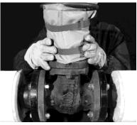
straps so as to tighten the Cut'n Wrap blanket. If insulating a **flange**, you are done with that pipe component.
