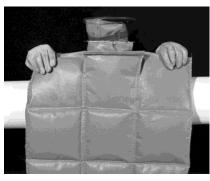
better fit on the pipe and around the valve stem. Wrap the valve blanket around one side of the valve stem, and then around the second side. Then come back to tighten the first hook and loop strap. You should loosen the hook and loop strap holding the second blanket in place so as to secure part of the third blanket around the valve stem.
