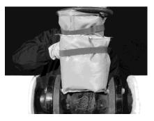
Inspect the insulated component to make certain that all bare surfaces have been covered with Cut 'n Wrap.
