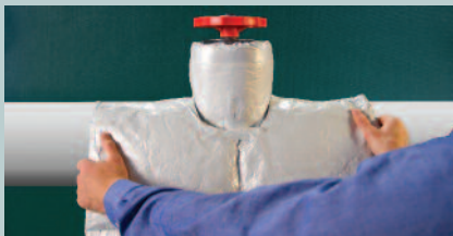
5. Repeat to Cover Additional Areas
