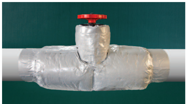
Figure 13 — Finished insulation. All seams are tightly sealed with tape and penetrations are tightly sealed with silicone caulk
