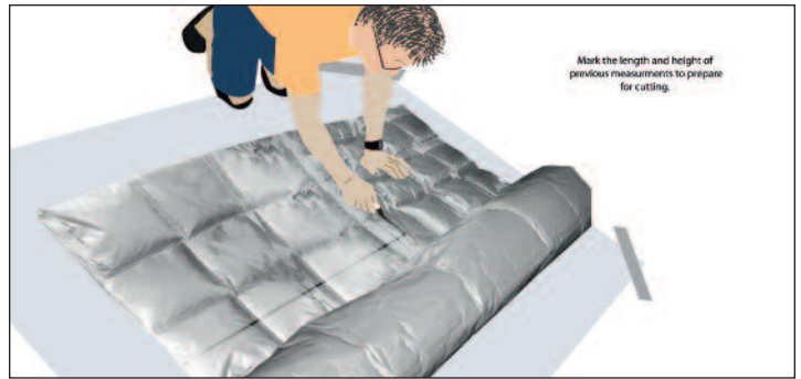
Figure 3 — Marking blanket to indicate cuts
