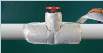
6. Tape to Pipe/Equipment and Seal any Openings with Supplied Caulk
