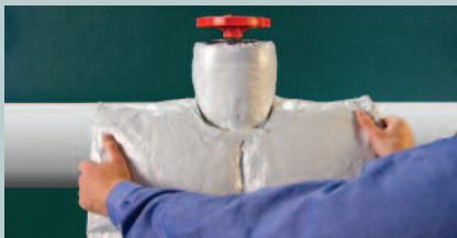
5. Repeat to Cover Additional Areas
