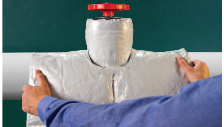
Figure 8 — Wrap blanket around fitting
