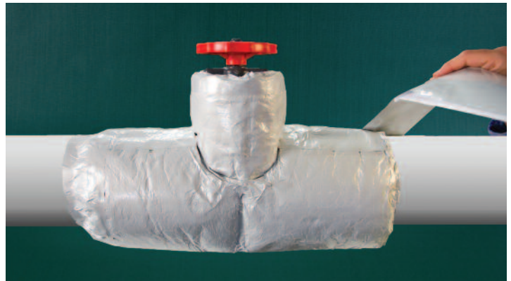
Figure 10 — Tape vertical and circumferential seams
