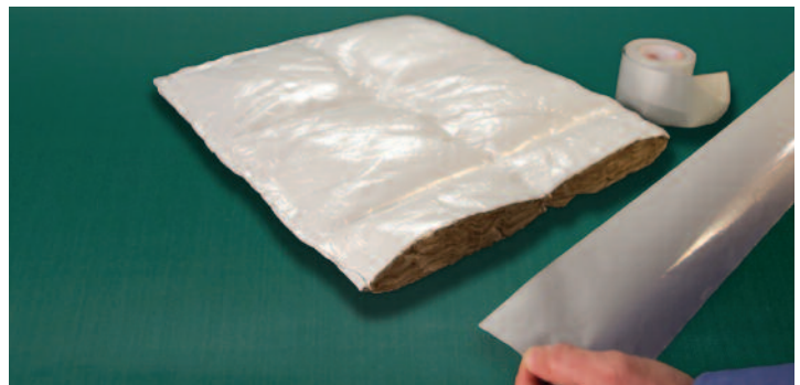
Figure 5 — Taping exposed blanket edge
