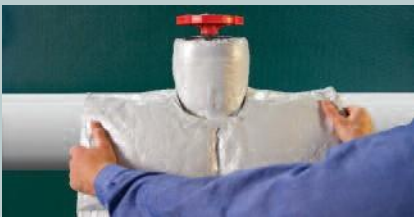
5. Repeat to Cover Additional Areas
