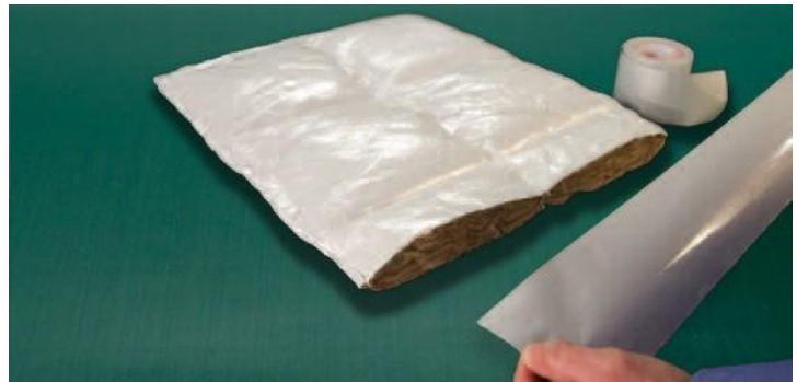
Figure 5 — Taping exposed blanket edge
