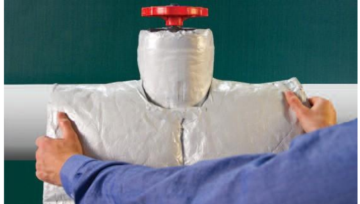
Figure 8 — Wrap blanket around fitting
