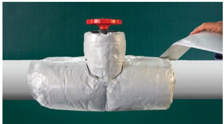
Figure 10 — Tape vertical and circumferential seams
