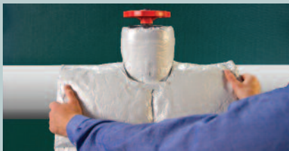
5. Repeat to Cover Additional Areas
