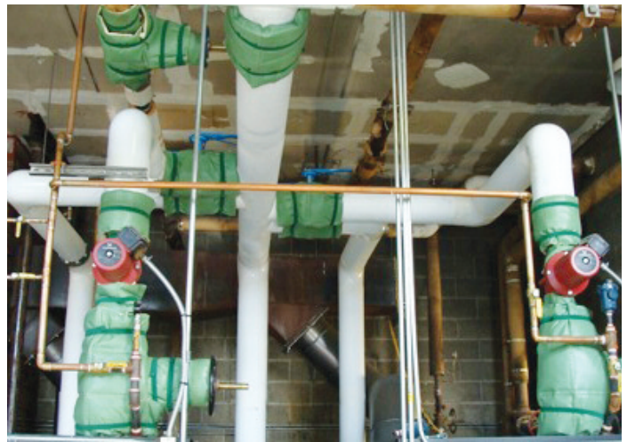
Ever Green Cut 'n Wrap blankets were installed to reduce the heat loss from the uninsulated valves and fittings on the University's forced hydronic system.
