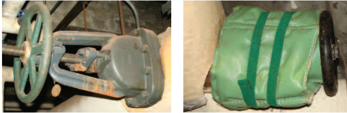
Figure 1A (on the left) shows a bare 4 inch NPS gate valve stem and Figure 1B (on the right) shows a similar gate valve stem insulated with an Ever Green™ Cut 'n Wrap™ insulation blanket. This single blanket on a 4 inch NPS gate valve stem is estimated to save about $45 per year of lost heat and reduce greenhouse gas emissions by about 530 pounds per year. The Cut 'n Wrap materials are estimated to cost about $38 for each of these valve stems.
