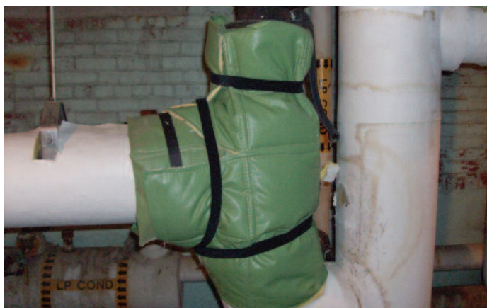
A pressure relief valve in CMMC's mechanical room insulated with a new Ever Green™ Cut 'n Wrap™ blanket.
