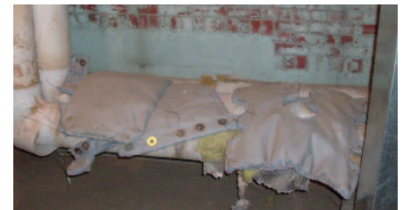
Many times custom made insulation wraps never get re-installed after maintenance work has been performed.
