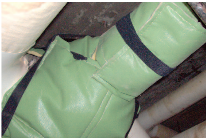
Another valve insulated with Ever Green™ Cut 'n Wrap™ insulation in the mechanical room at CMMC.
